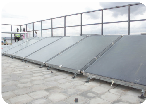
Water heating solar panels
